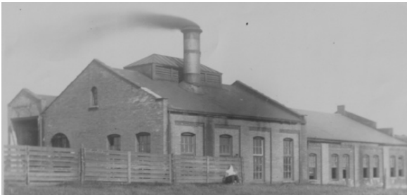
Power house north of Lima. (courtest, Doug Morgan)
